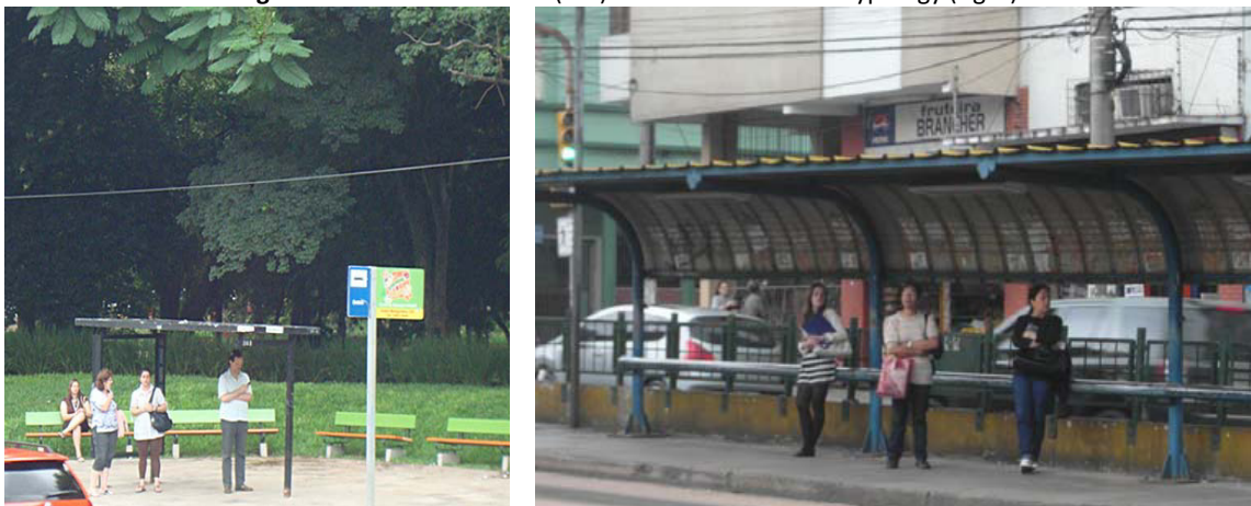
Figure 25 – Park bus shelter (left) and bus lane shelter typology (right)
