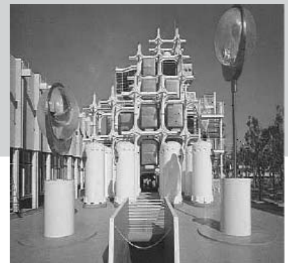
FIGURA 1.9 NORIAKI KUROKAWA, PAVILHÃO TAKARA BEAUTILLION, OSAKA, 1970
