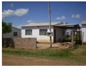
(b) Moradia na Rua Bugre Lope
