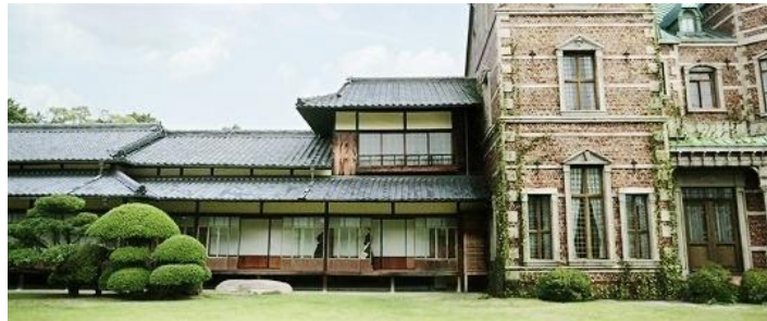
Figure 2 - Japanese wing and British wing of the mansion
