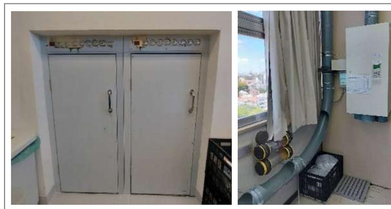
**Figure 13** - Left: elevator that connects the main hospital warehouse to the ICU pharmacy; right: pneumatic tube and capsules for placing materials.
