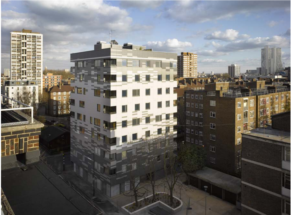
Figure 1.1 – Stadthaus Building in Murray Grove Street, London. (Wood Skyscrapers, s.d. ).
