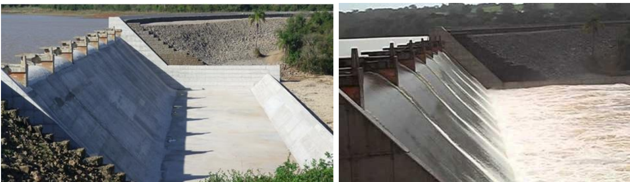
Figure 12.- Ernestina Hydropower Plant, Brazil. Left: empty stilling basin. Right: hydraulic jump.
