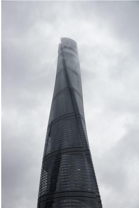
Figura 7 – Shanghai Tower (Xangai, China)
