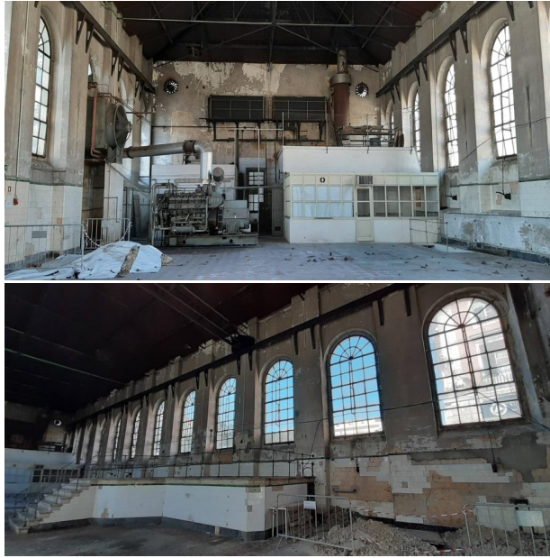
Figure 5: Internal views. Power plant. HCB. Lisbon. Source: the author.
