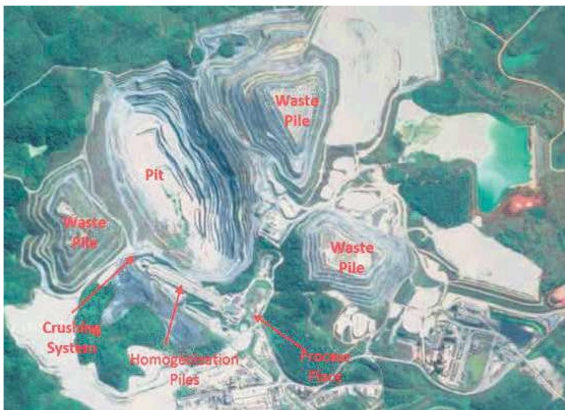
Figure 2 - Overall view of the pit location and the surrounding surface structures
