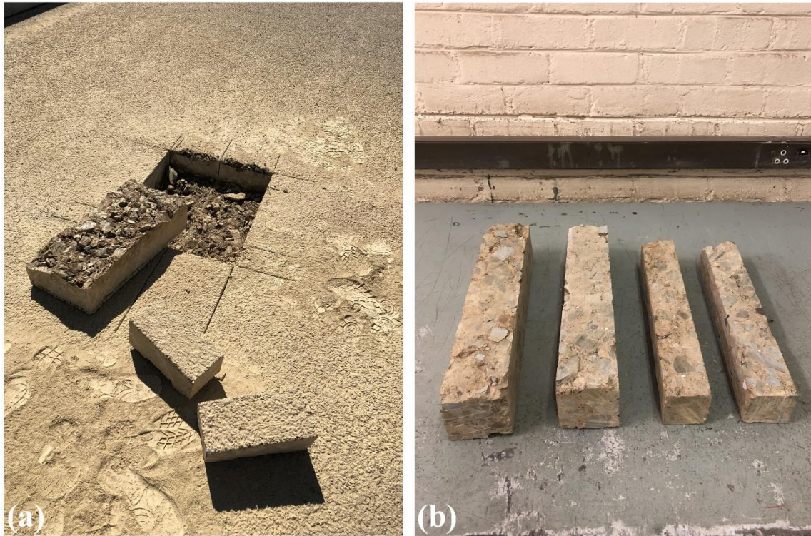
Figure 3. Field specimens: (a) slabs taken from the LCSM; and (b) beams cut from a slab
