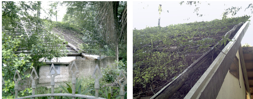
Figure 3.5: Green roofs oriented to the South (a) with significant areas without plant coverage; and (b): with insufficient plant coverage. (Krebs, 2005)
