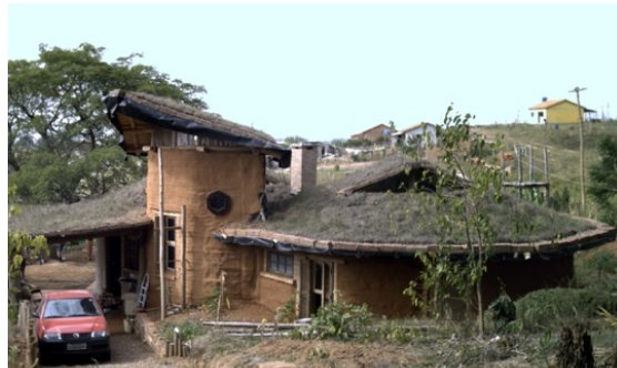
Figure 3.3: Complex self-constructed green roof (Krebs, 2005)
