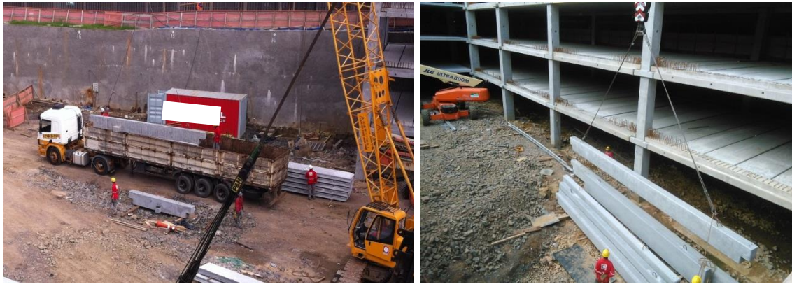
Figure 5 - Lifting of beams
