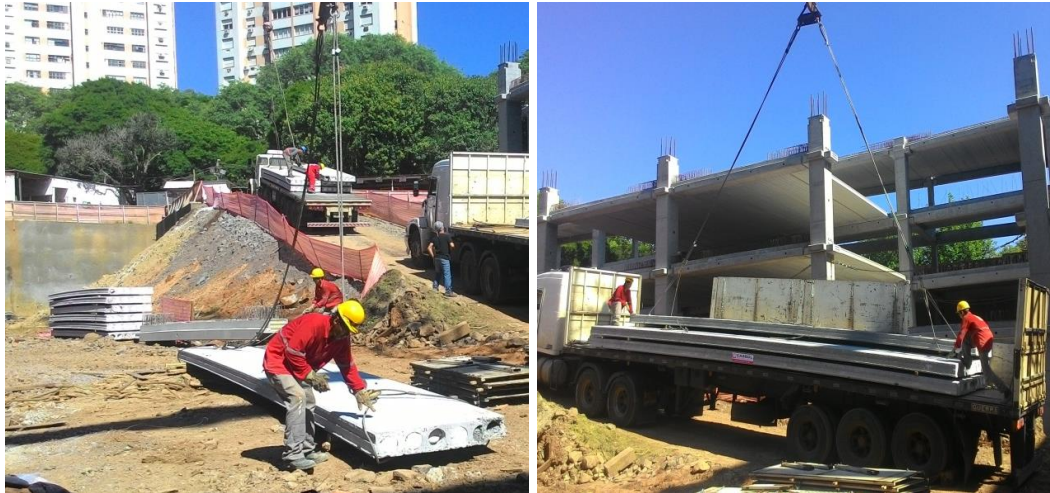
Figure 12 - Lifting and handling a slab
