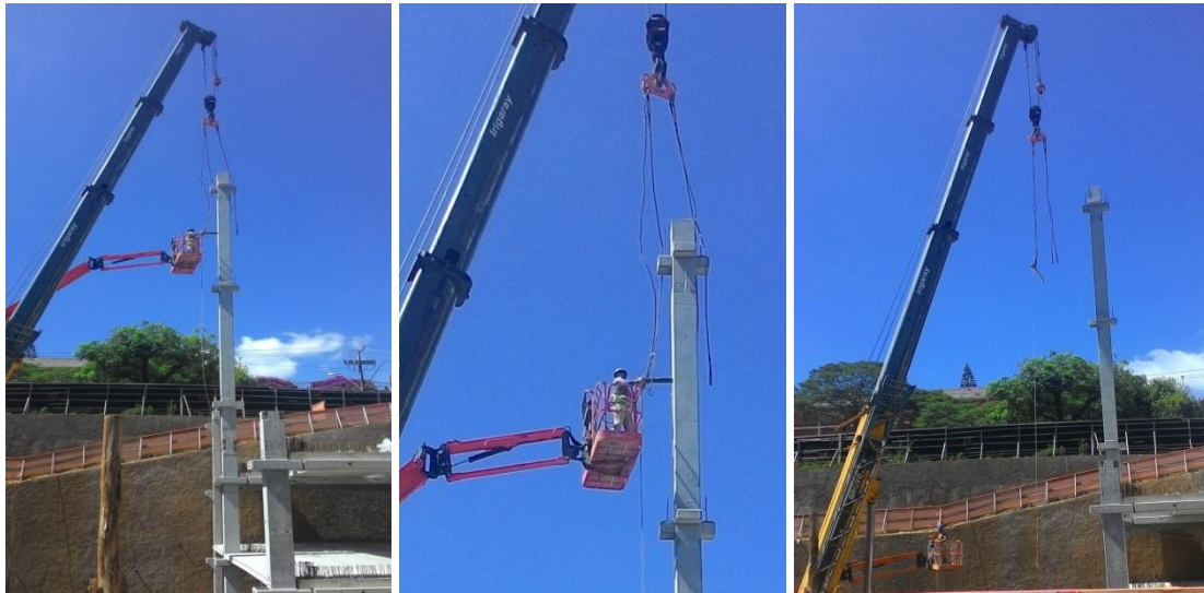
Figure 11 - Experienced assembler removing the lifting pin
