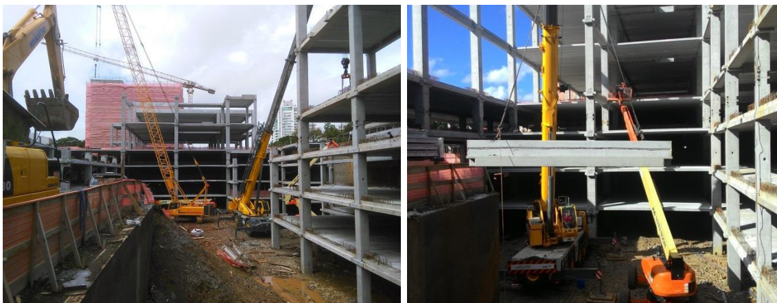
Figure 6 - Restricted space to maneuver equipment and handling components
