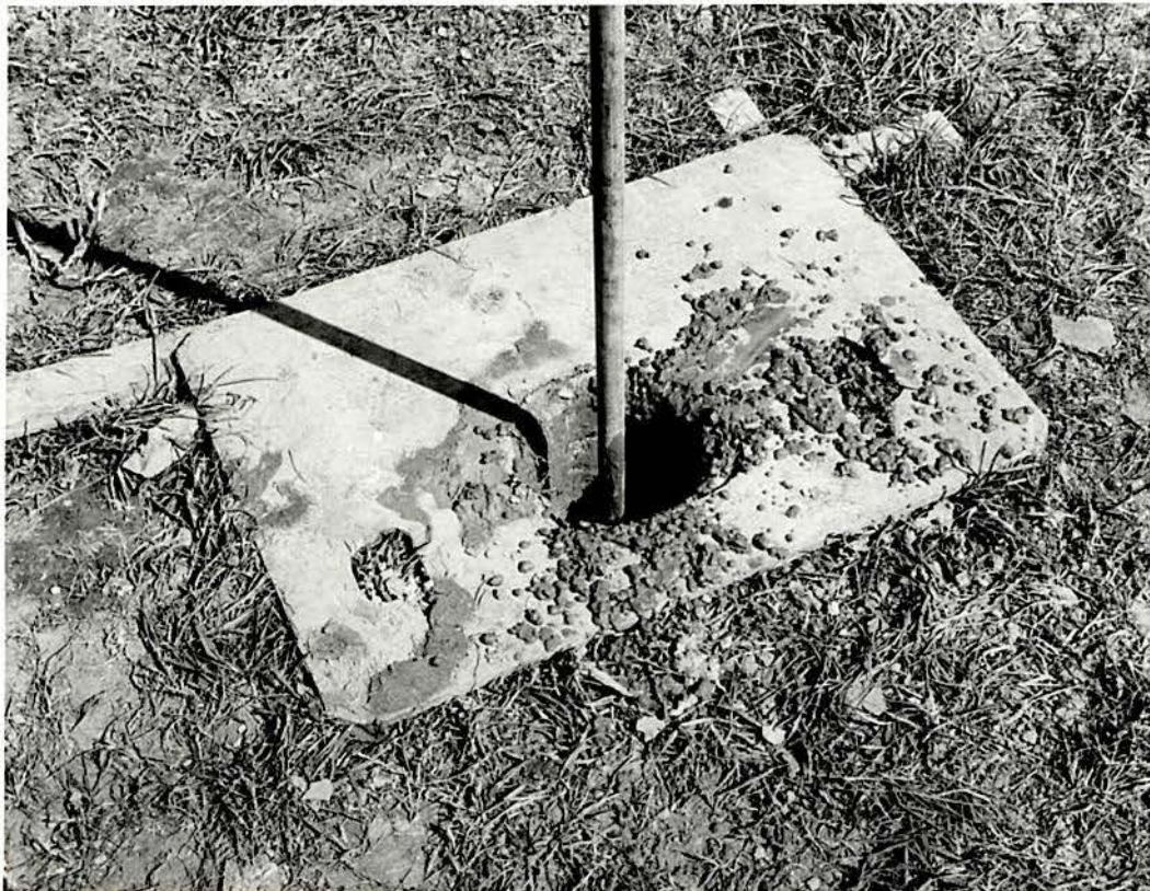
(B) Detail of the model pile installation (New pressure cell in position)
