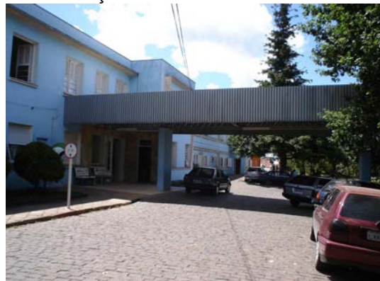
Acesso Principal Hospital
