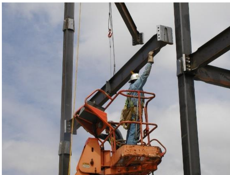
Figure 7.34: A worker placing the beam in the correct place
