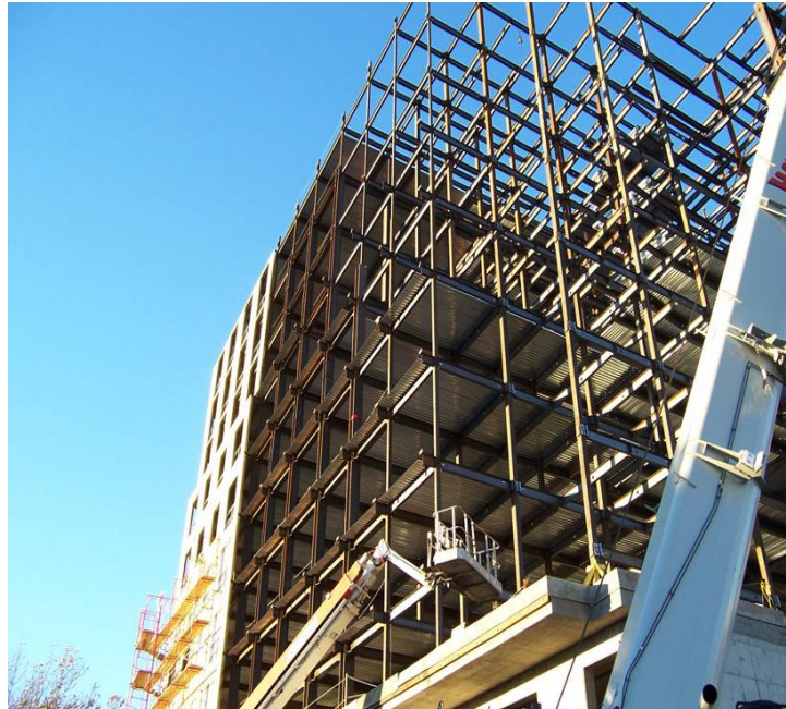
Figure 7.33: Example of the erection process
