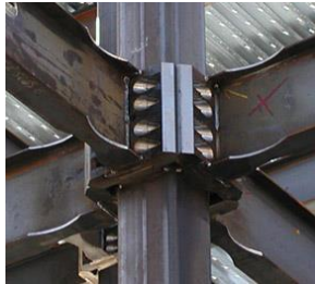
Figure 7.25: R-type connection
