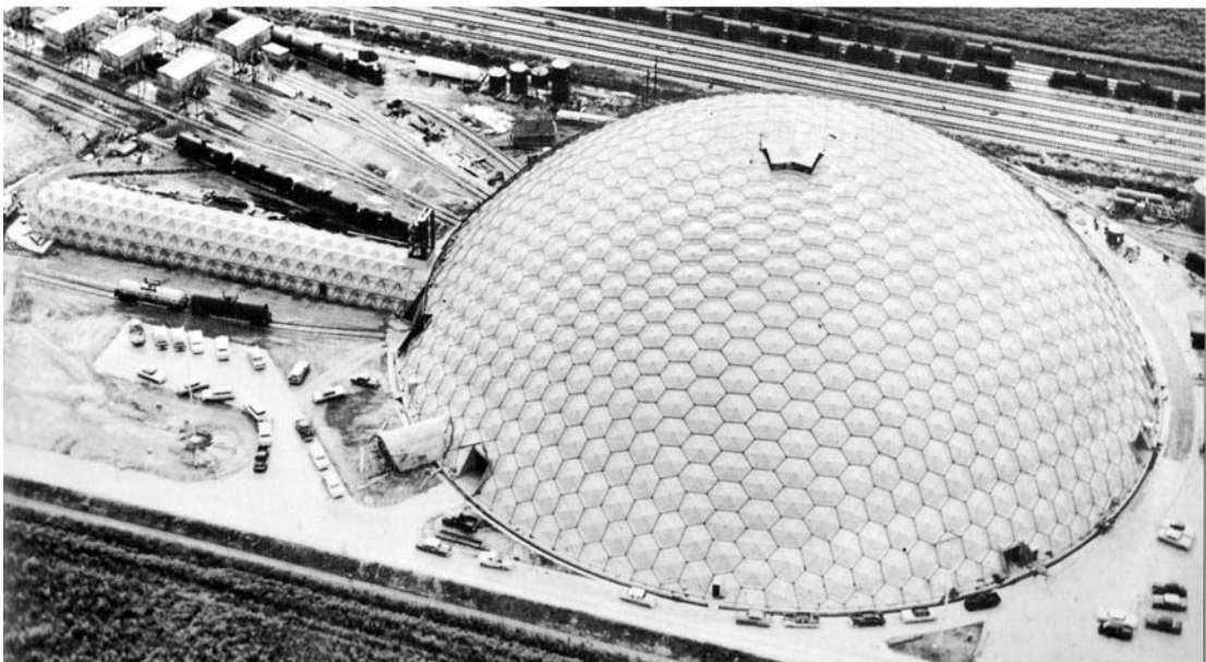
8 - DOMUS GEODÉSICO PARA A UNION TANK CAR COMPANY BATON ROUGE, LOUISIANA, 1958
