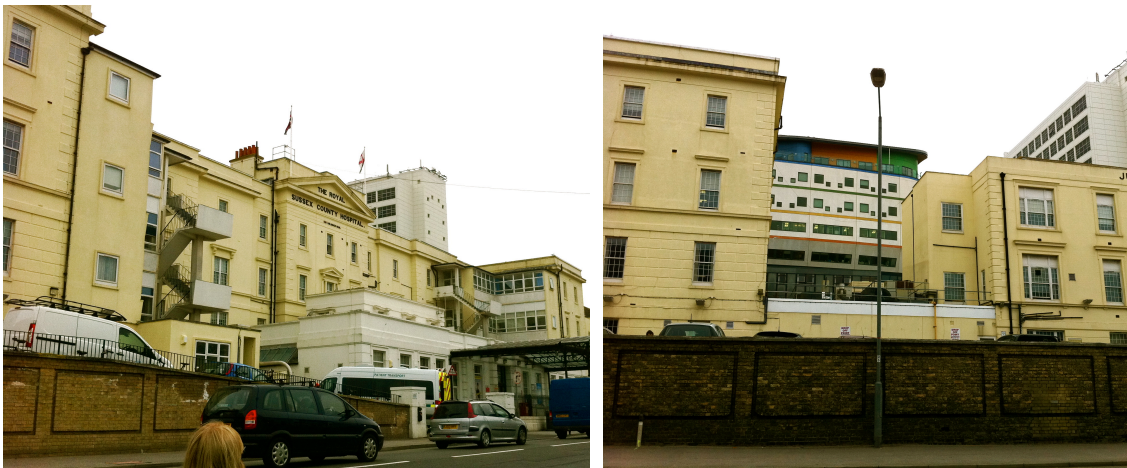
Figure 34: Barry and Jubilee Buildings
