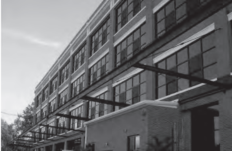
4 [anexo 28] Reynolds Lofts Louisville/KY, 2005
