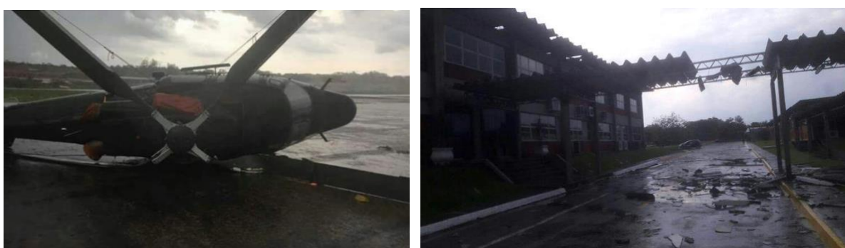
Figure 4.20 – Photo of damage caused by strong gusts at SBTA – Taubaté Airforce Base, SP, 27/10/2017 (Source: O Vale)
