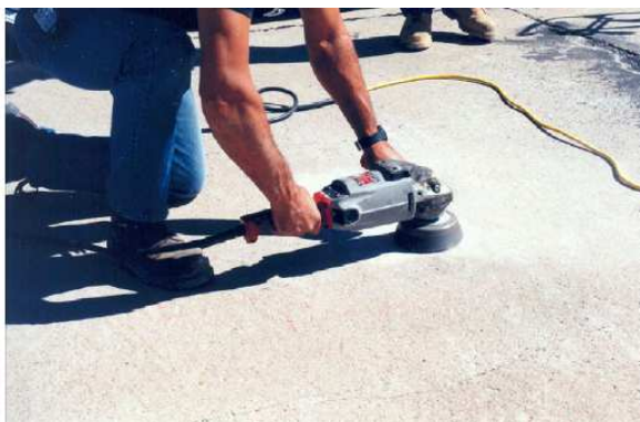
Figura 3.3 - Lixamento Mecânico (Wyoming Department of Transportation, 2006)
