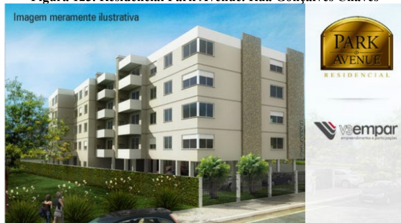
Figura 123. Residencial Park Avenue. Rua Gonçalves Chaves
