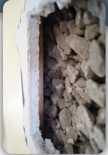
Parede no-fines observada in loco
