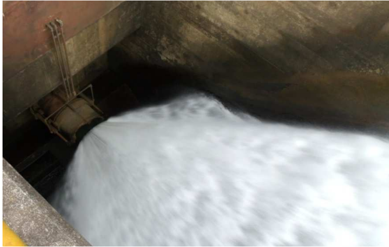
Figura 5-7 – Válvula dispersora Rowell DN600 mm.
