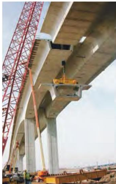
Figura 2.9 - Ponte Victory ( http://www.asbi-assoc.org/news/project/index.cfm?aid=274 )
